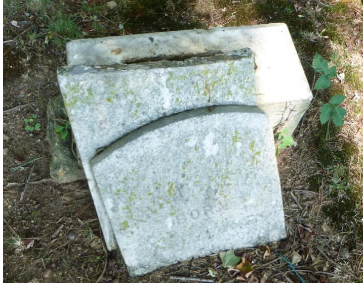
Repair break and reattach to base
