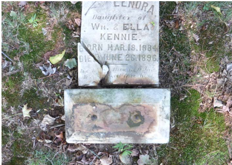
An example of the failure of iron pins.
