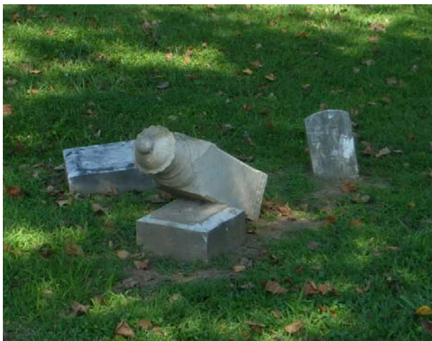
An example of an obelisk that needs to be reset on a leveled base.
