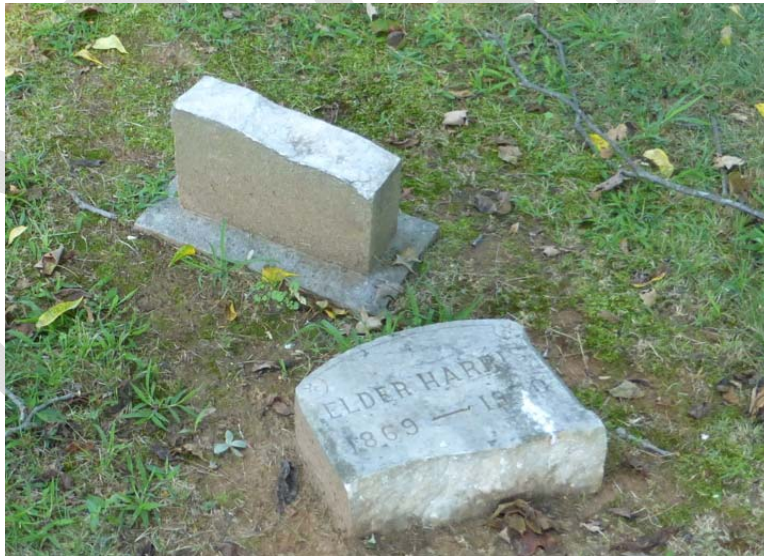
The Elder Harris gravestone is an example of a simple break that should be repaired.
