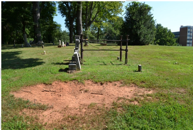
There are also additional areas of the cemetery that require erosion control treatment.
