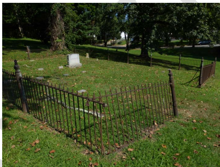
Cast iron enclosure.
