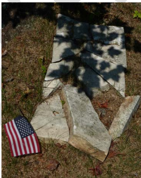
An example of a gravestone where there is an immediate need to reattach multiple fragments and reset.
